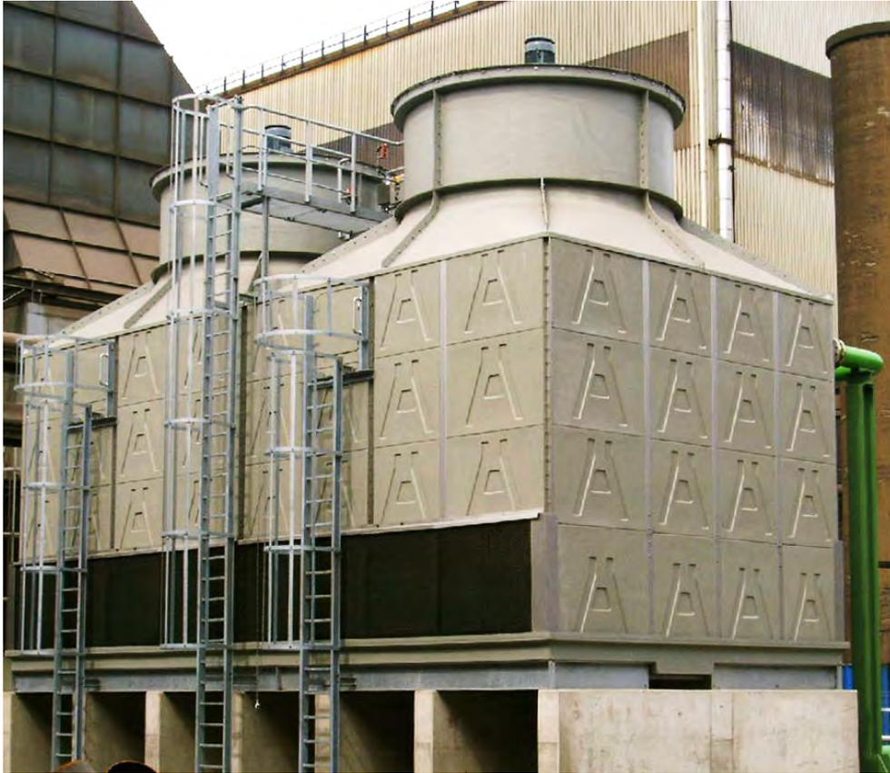
**CP** towers are induced draft, stainless steel structure with fiberglass cladding, counterflow cooling towers, designed to serve light to medium industrial process loads on clean and dirty water. For more than 30 years the CP continues a reputation of high reliability and low sound even when operating in high temperature, high wind load environments. The CP can be shipped and lifted preassembled or on larger models, preassembled into modules for final assembly at site.
